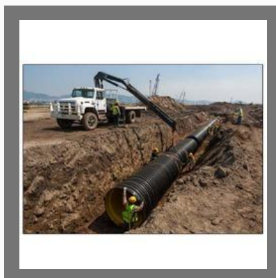
HDPE Pipe Installation Services
