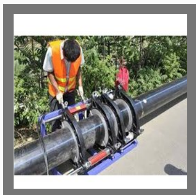
HDPE Pipes Welding
